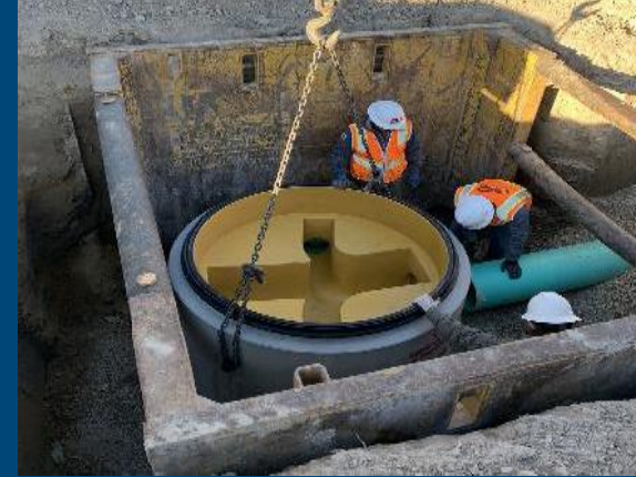
Lined RCP Pipe & Manholes
