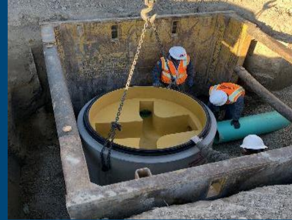
Lined RCP Pipe & Manholes
